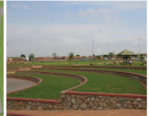
Fig 31 Amphitheatre entrance ramp
